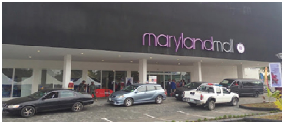
Fig. 2. Front view of Maryland shopping mall
